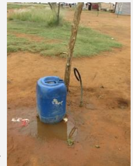
Shared water connection in Phumekhaya
