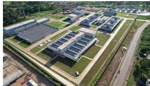
Drinking water treatment plant
