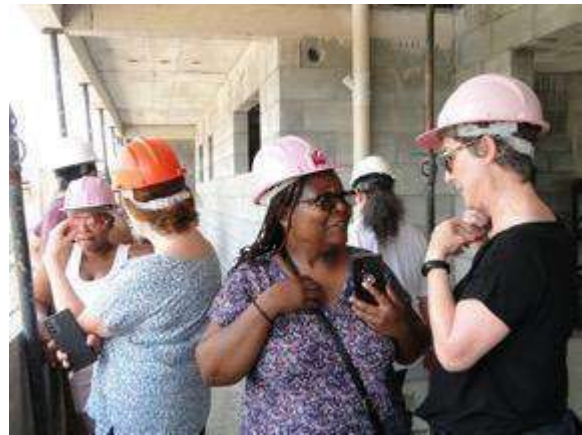
Visit to the Carolina Maria de Jesus Mutirão construction site. Photo: Paula Freire Santoro, 13 March 2024.
