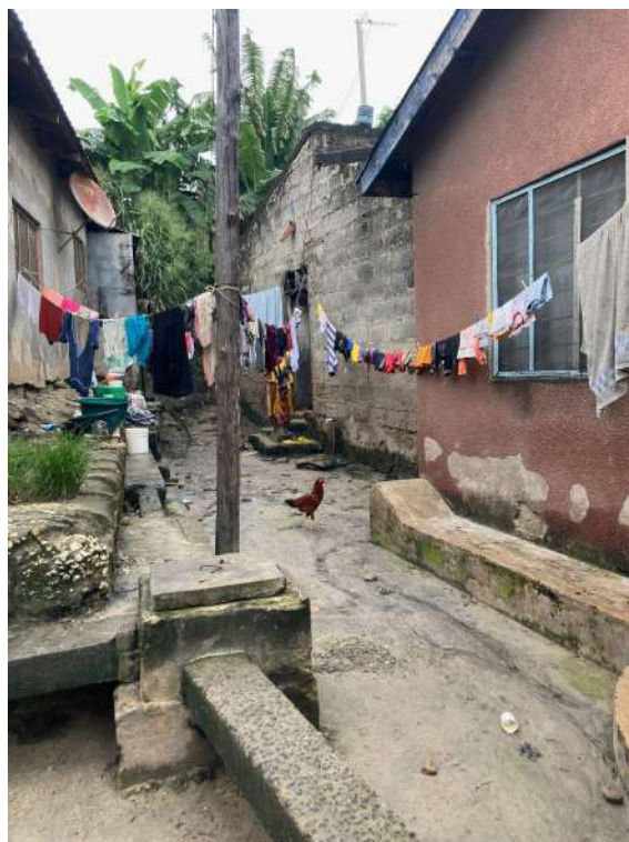
Elements of the simple sewage and biogas generation system. Vigunguti, Dar es Salaam. Photo: Priscila Izar, 19 April, 2024.
