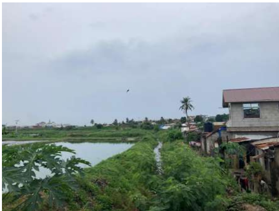
The Vigunguti informal settlement borders one of DAWASA's treatment ponds. Vigunguti, Dar es Salaam. Photo: Paula Santoro, 19 April, 2024.
