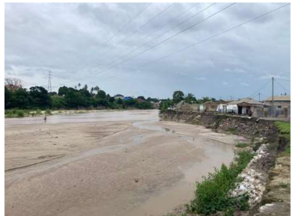
The Msimbazi river in Karakata, a hazardous area where in January 2024 over 60 families lost their homes due to flood-related damages. Karakata, Dar es Salaam. Photo: Albert Nyiti, 19 April, 2024.
