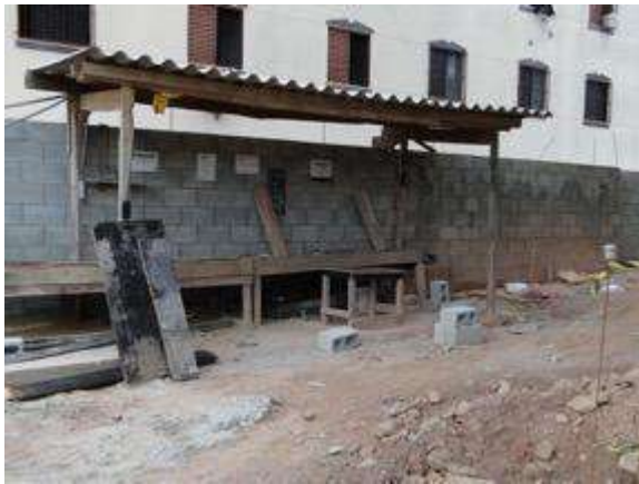
Mutirão Dandara construction site. Photo: Amanda Silber Bleich, 15 March 2024.
