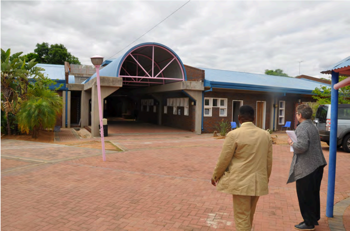
Fig 6.28: University of Mpumalanga Siyabuswa Campus renovation of the existing offices, library and lecture venues.
