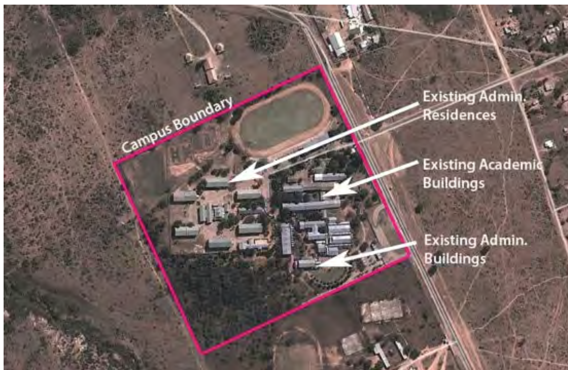
Fig 6.16: Aerial Image of the existing Siyabuswa Campus indicating the existing Buildings, which were renovated during from 2012-2015.
