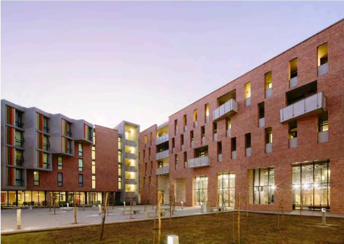
Fig. 12.5: Sol Plaatje University Campus Building 01. View of the Internal Courtyard (T. McLaren)
