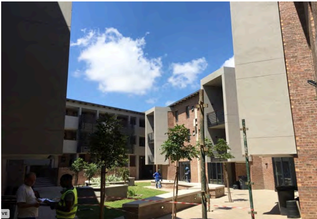
Fig 13.21: University of Mpumalanga Campus Building L007. The NU PMT oversaw the design of the building, and UMP its construction.
