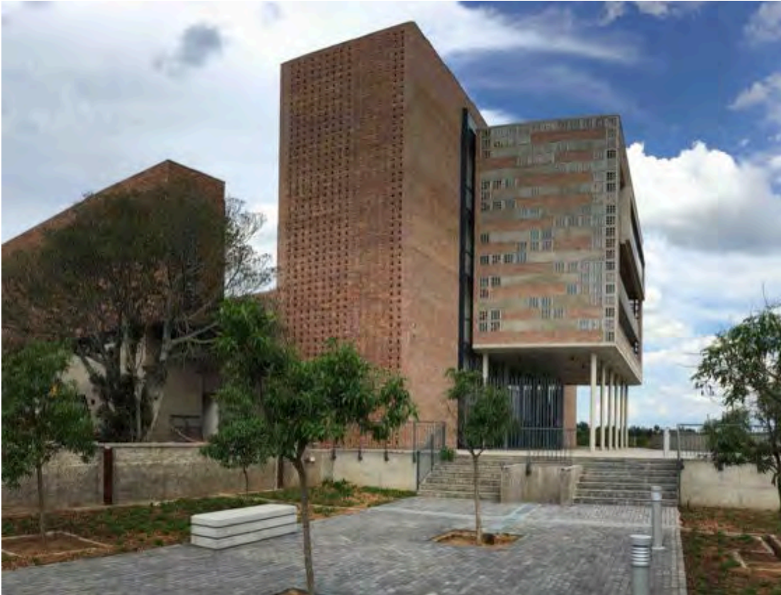
Fig 13.14: University of Mpumalanga Campus Building L02 – Executive Office Building. Building accommodates the university executive, boardrooms, dining amenities and council chamber. The NU PMT oversaw the design of the building, and UMP its construction.
