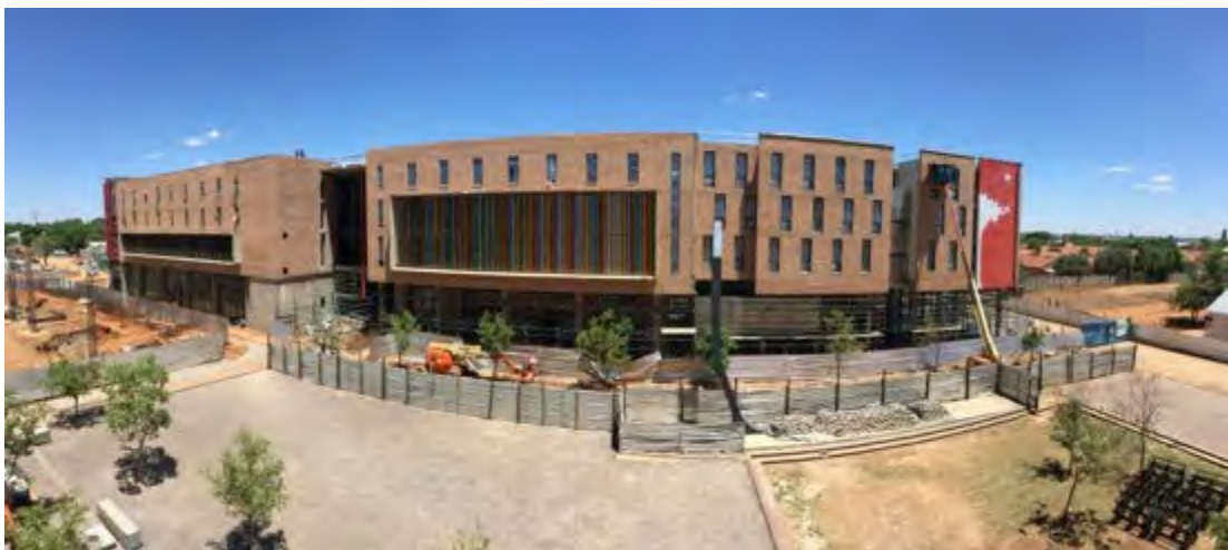
Fig 10.3: Central Campus Square Sol Plaatje University as focus for surrounding academic and residential buildings.
