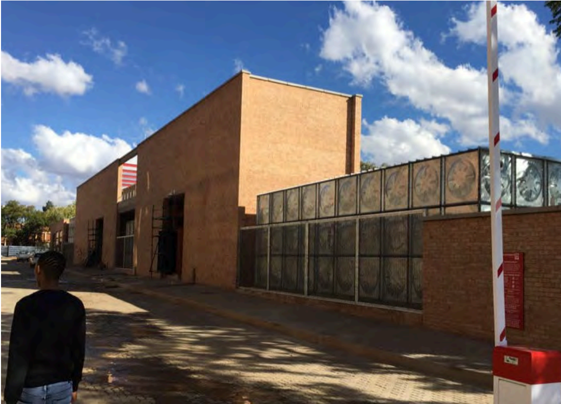
Fig 12.14: Sol Plaatje University Campus Central Services Building. Most bulk services, waste management, water supply and electrical back-up for the 1 st two phases of construction located in the Central Services Building.
