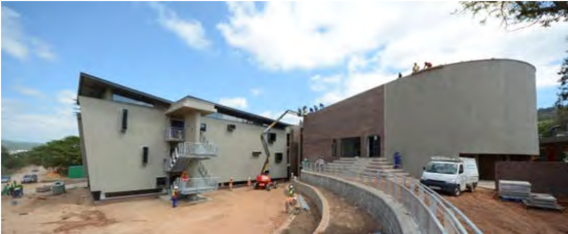
Fig 10.10: Auditorium and Library building within the Science Block at the University of Mpumalanga
