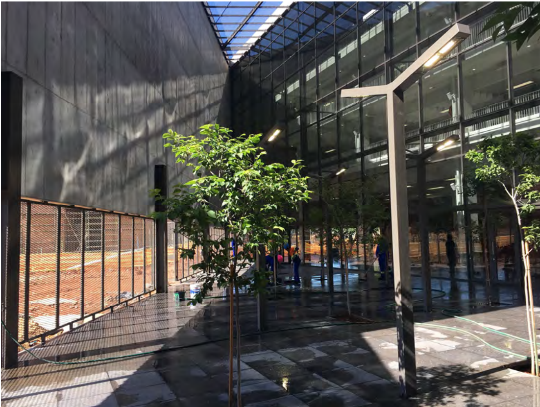
Fig 12.13: Sol Plaatje University Campus Building 04. The Internal Courtyard
