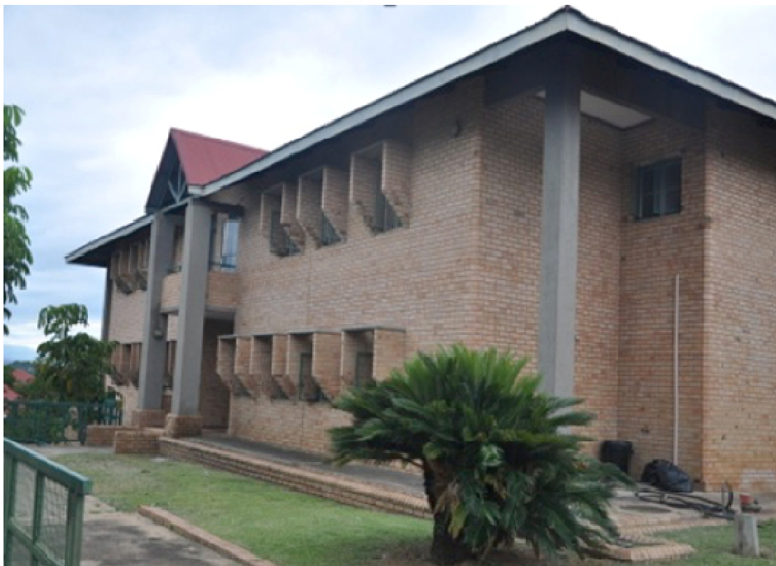
Fig 6.27: University of Mpumalanga renovation of the existing five residence buildings.
