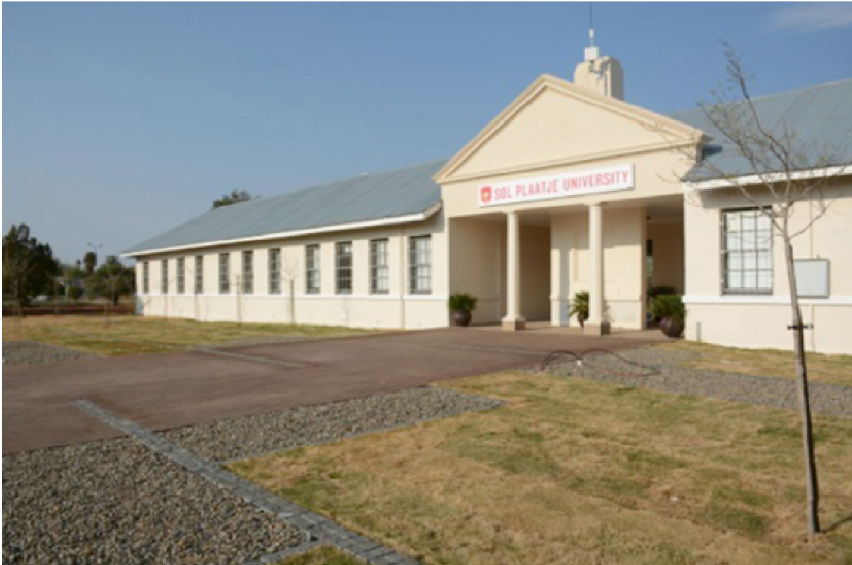
Fig 7.4: SPU changes to the historical William Pescod School. Entrance changed to allow access through to the Central Campus.
