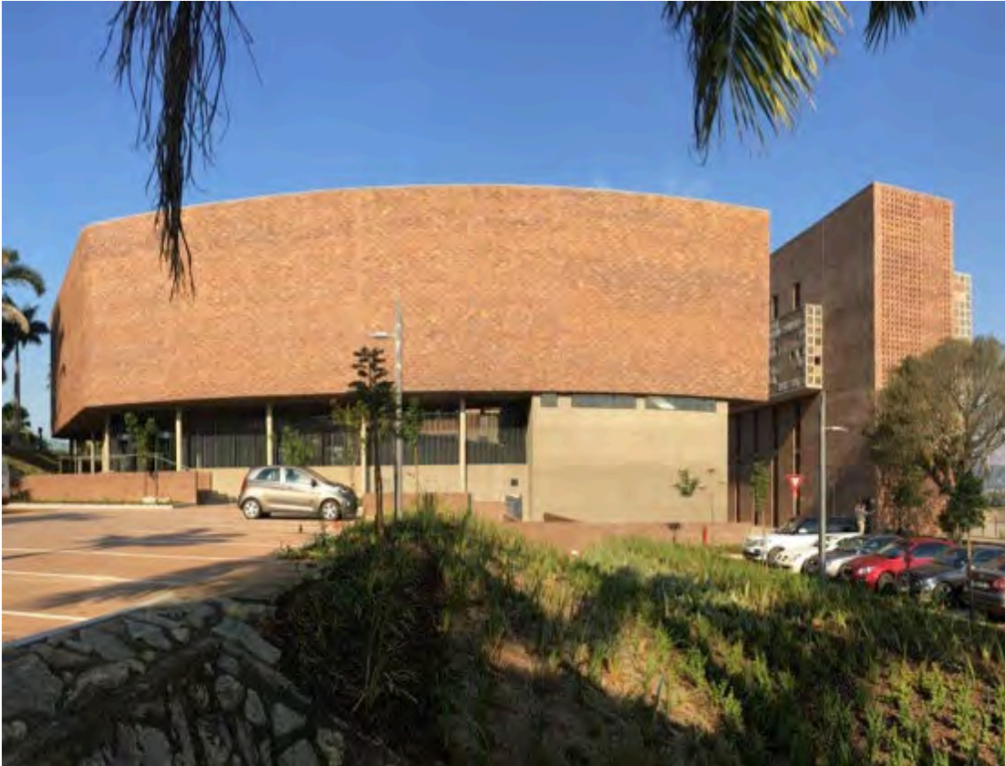
Fig 13.16: University of Mpumalanga Campus Building L03 – Library and Student Resource Centre. Building sits behind the Executive Office. The NU PMT oversaw the design of the building, and UMP its construction.
