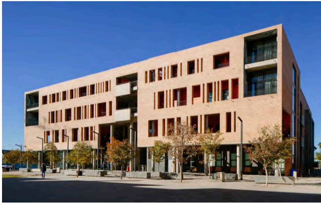
Fig 12.9: Sol Plaatje University Campus Building 03. The first new academic building with multiple seminar and lecture venues, four raked auditoriums, staff offices, student support and campus retail on the ground floor facing the central campus square.
