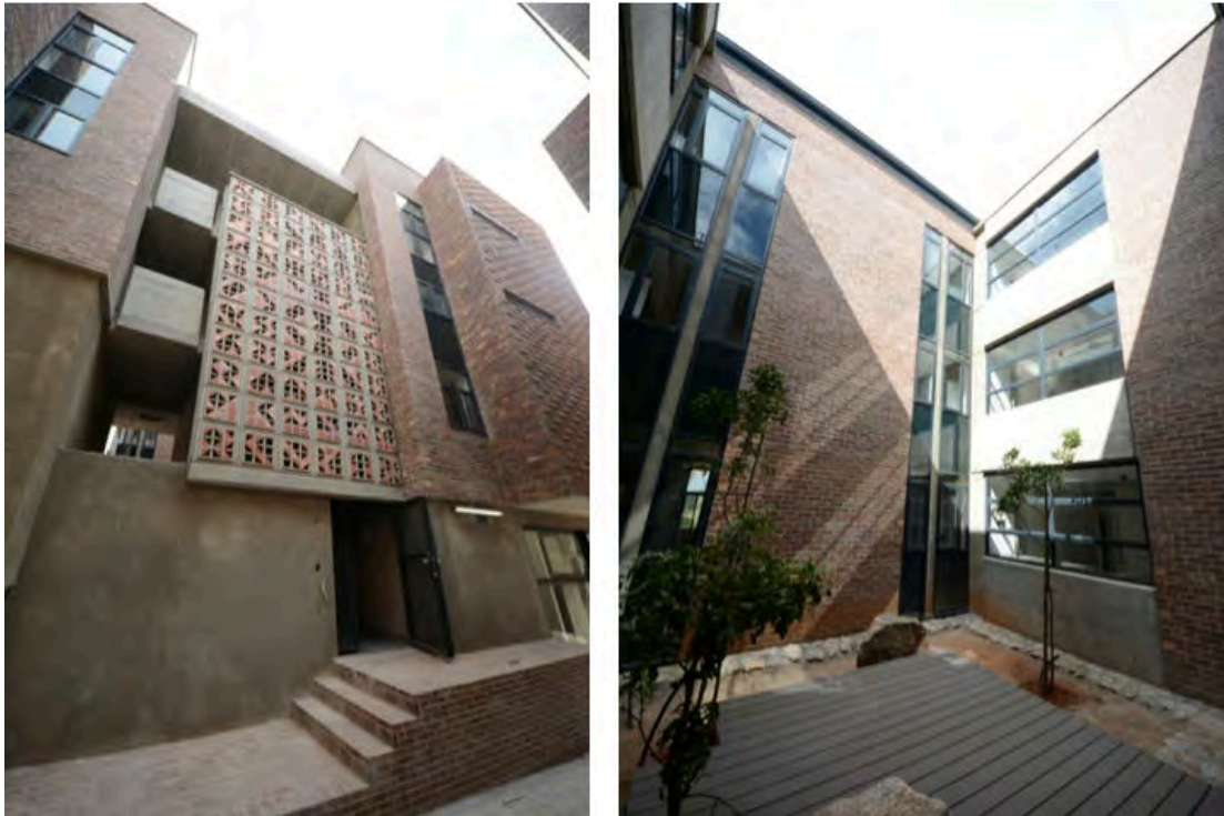
Fig 13.4: University of Mpumalanga Campus Building L001 – Student Residence. Building accommodates 238 students, Game Rooms, Laundry, study spaces and seminar rooms. View of Residence Courtyards
