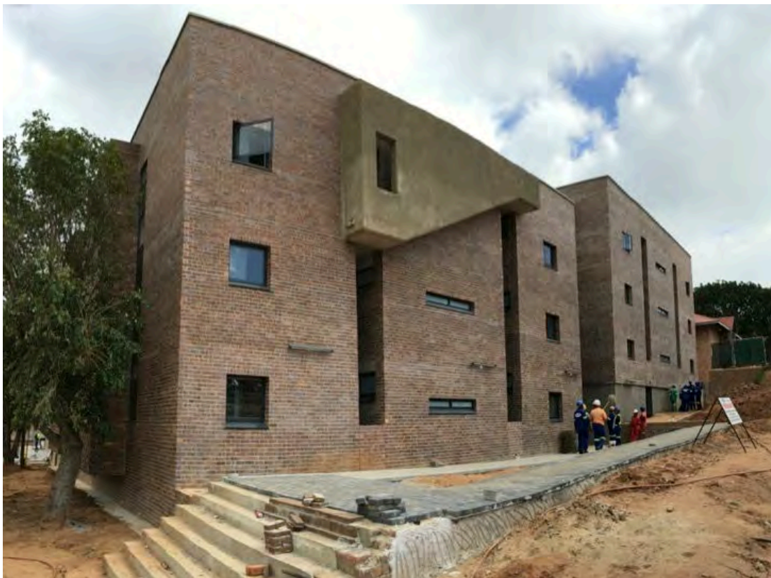
Fig 13.5: University of Mpumalanga Campus Building L001 – Southern façade facing the campus entrance gate.
