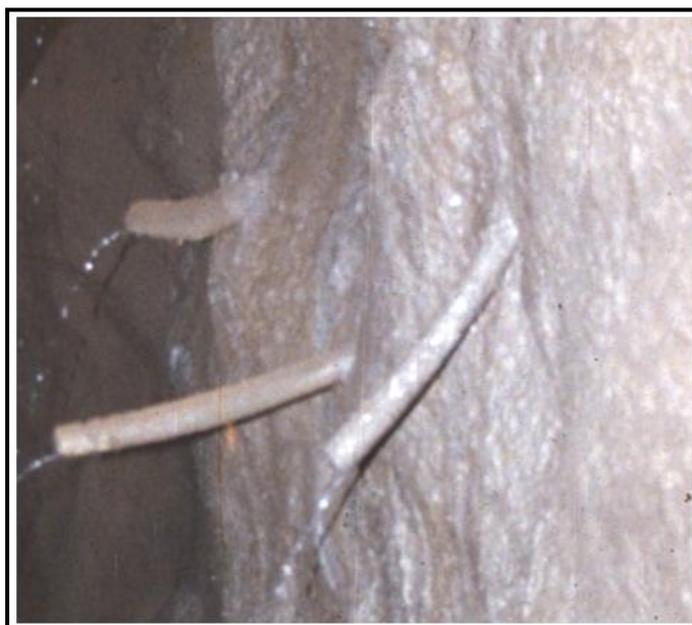
Figure 2. 7 Plastic fitted drain holes After (Hoek, 2011)
