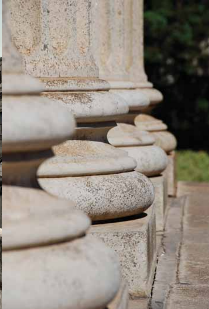
William Martinson Central Block: Solid Foundations
