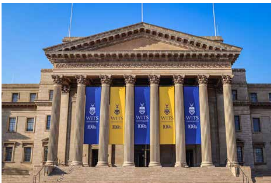
The restored Wits facade.
