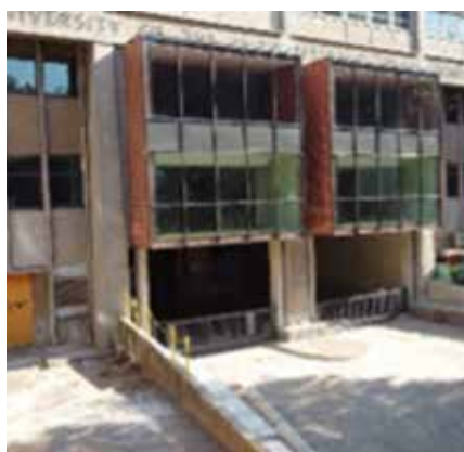
New insert across lower ground and ground floor levels of previous unlinked areas
