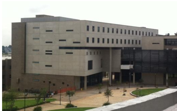
South west façade
