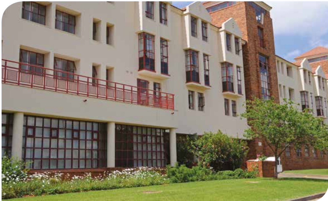
Barnato Hall Residence
