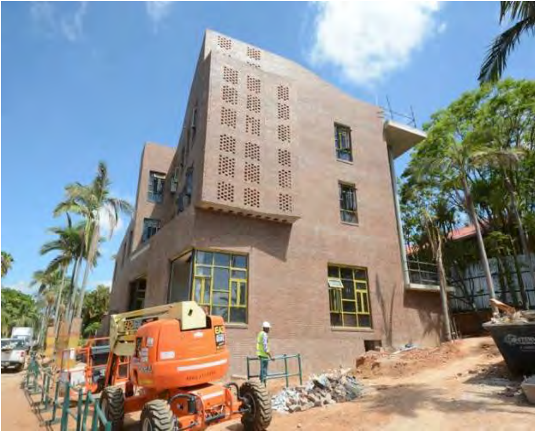
Fig 13.13: University of Mpumalanga Campus Building L04 – Administration Building.
