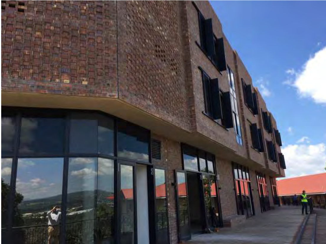
Fig 13.20: University of Mpumalanga Campus Building L07 – Residence, Student Wellness and Multi-purpose Hall Project. The building planned over two phases accommodates 140 student beds, a student wellness centre, gym and student union offices as well as a multi-purpose hall for 1000 people.
