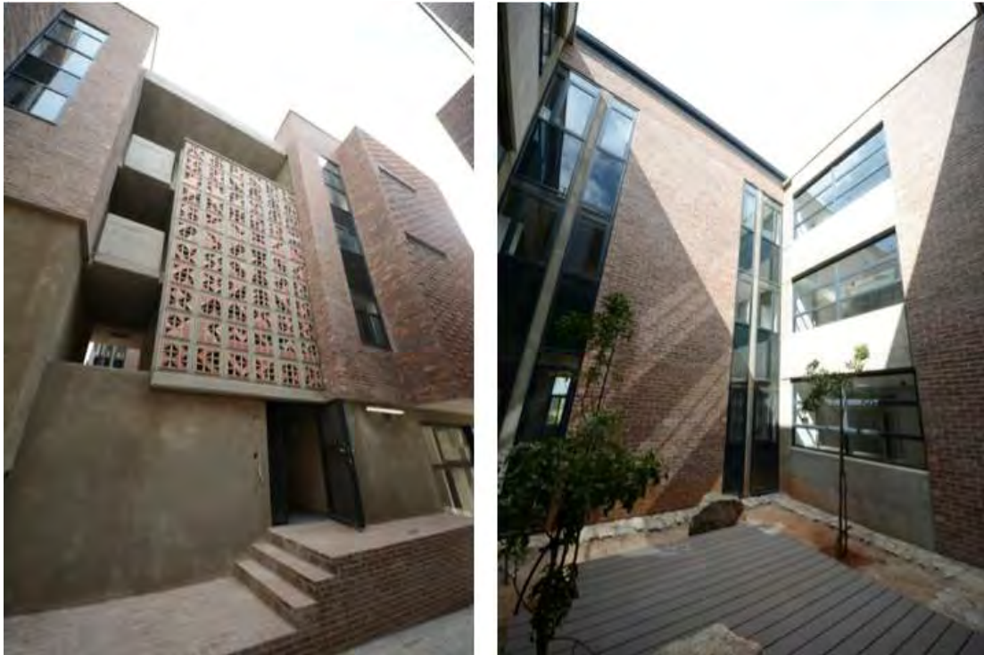
Fig 13.4: University of Mpumalanga Campus Building L001 – Student Residence. Building accommodates 238 students, Game Rooms, Laundry, study spaces and seminar rooms. View of Residence Courtyards
