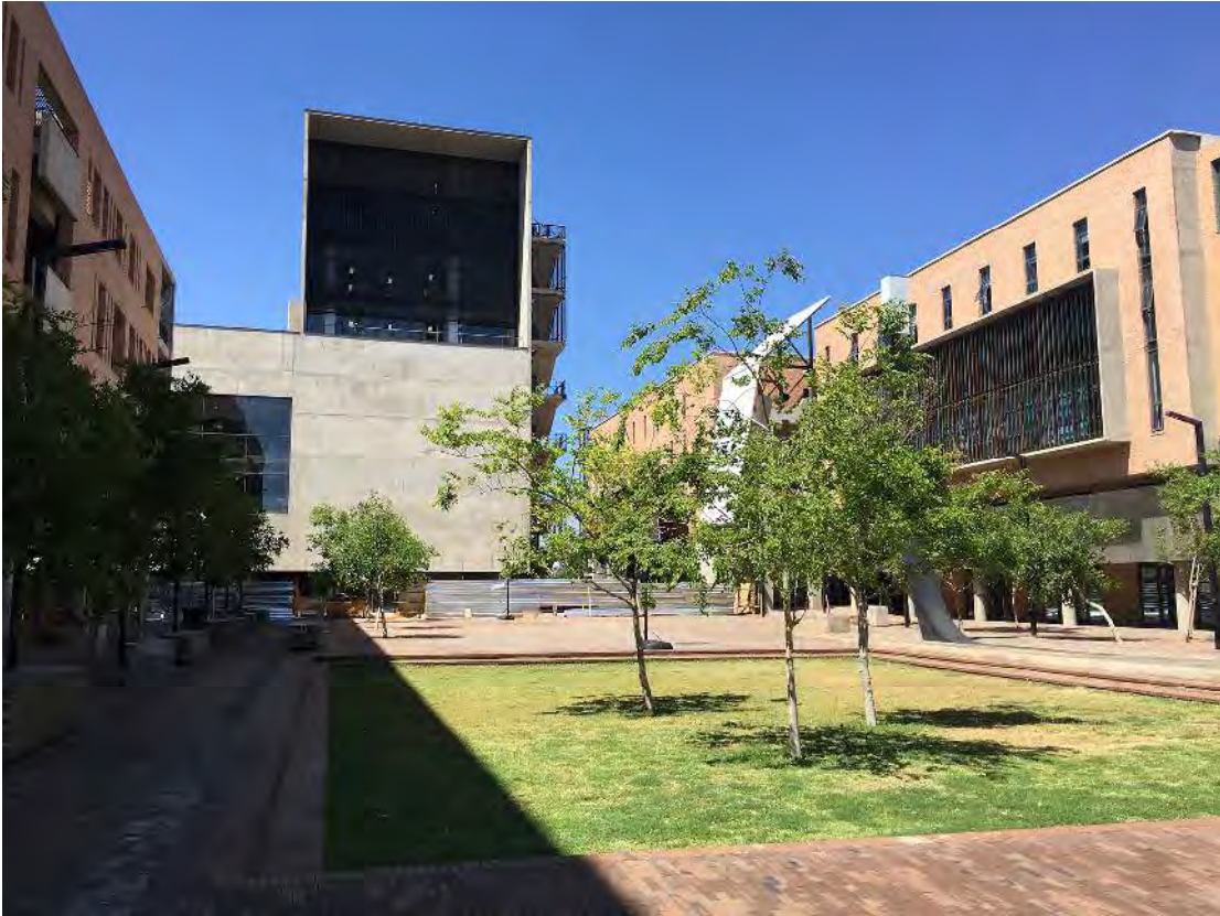
Fig 12.12: Sol Plaatje University Campus Building 04. Library and Student Resource Centre. Landmark building facing the Central Campus Square.
