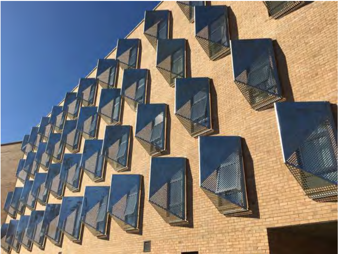
Fig. 12.7: Sol Plaatje University Campus Building 02. West facing residential façade, with sun screening elements.
