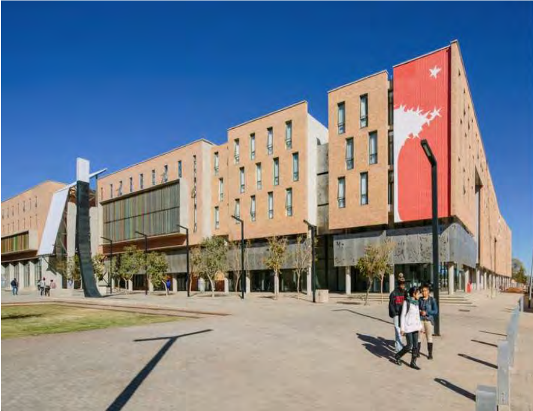
Fig 12.4: Sol Plaatje University Campus Building 01 on the corner of Scanlan Road and facing the Central Square. Residence for 290 students with retail, game rooms, seminar space, a laundry and the universities ICT facility.
