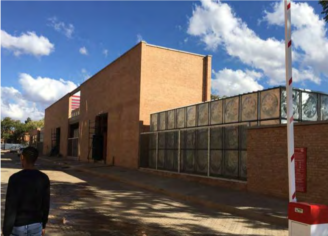
Fig 12.14: Sol Plaatje University Campus Central Services Building. Most bulk services, waste management, water supply and electrical back-up for the 1 st two phases of construction located in the Central Services Building.
